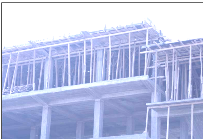
Poplar poles as used in a standard construction project in Kabul. Winter 2007. Photo: WCS, J. Wingard.
