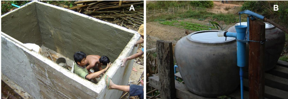
Figure 5.7.1. Cistern installation for water storage (A) and irrigation (B). Water management is a key component of adaptation to irregular precipitation patterns.
